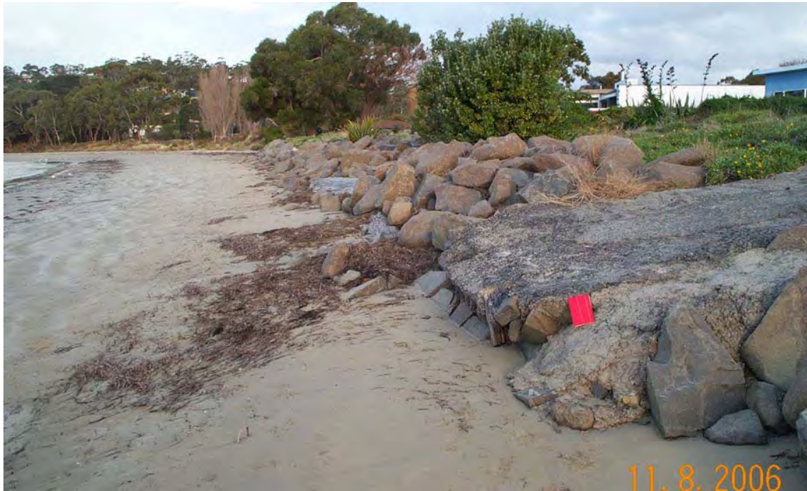
Figure 29: Photo RB2006_20 (Viewpoint 13). This view shows a concrete boat ramp in the boulder wall along part of the southern area of Roches Beach. Lowering of the beach surface below the lip of the ramp is probably a result of recent stormy conditions. The surface will probably grow (accrete) upwards during long calm weather periods, however it is likely that some degree of net lowering of the beach surface has occurred since the boulder wall was constructed in 1988, due to increased wave reflection off the hard wall. Red notebook is 180mm high.
