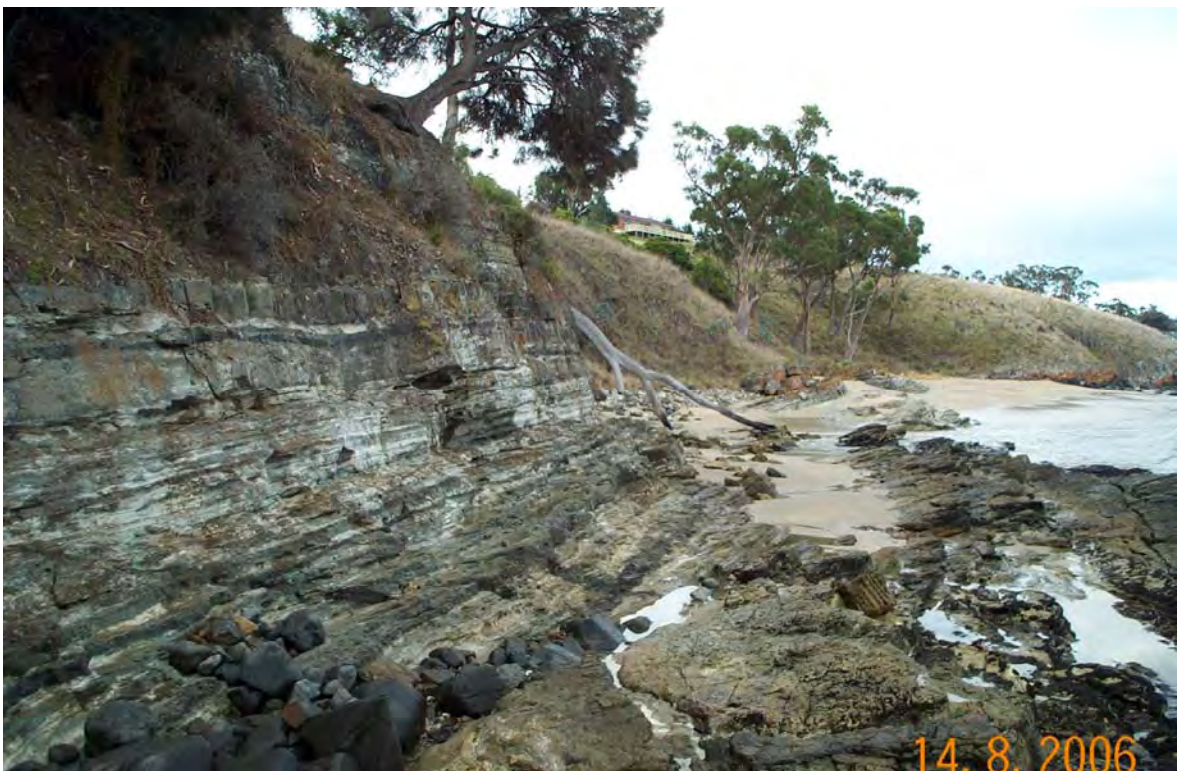
Figure 36: Photo RB2006_103 (viewpoint 53). View north along part of the northernmost end of Roches Beach, where the beach is backed by a rising bedrock slope with little dune development. There is little potential for shoreline recession here, although beach lowering and loss may result from sea level rise.
