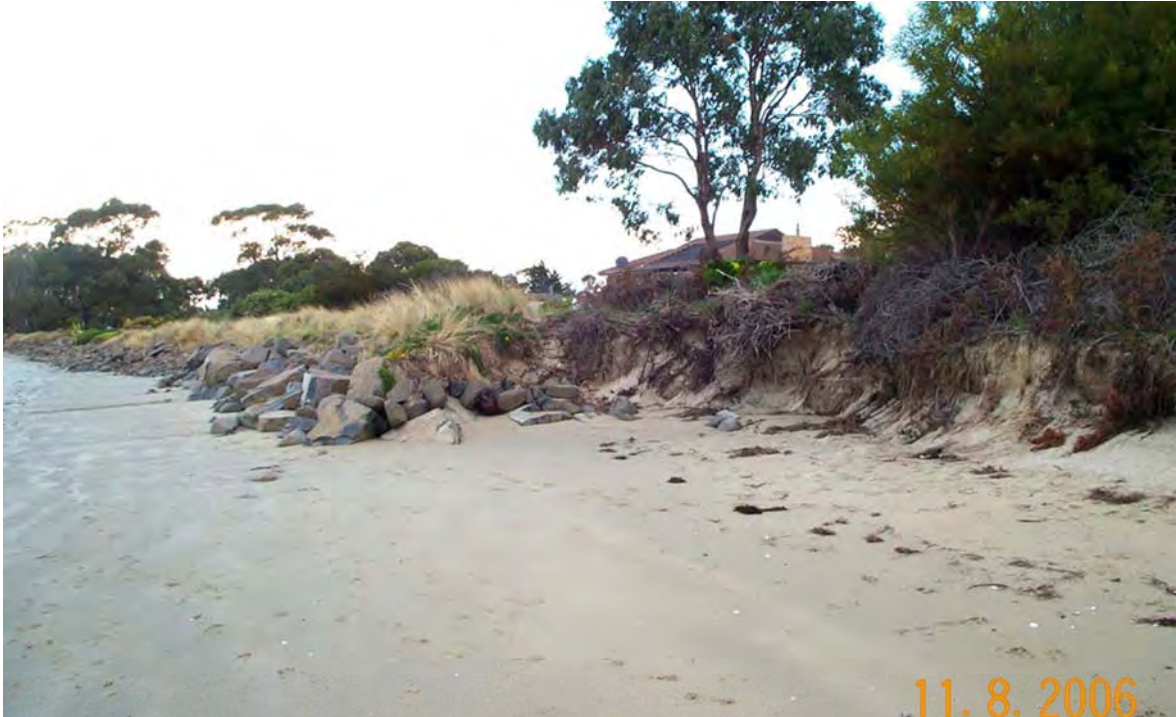
Figure 31: Photo RB2006_28 (Viewpoint 17). View southwards from the northern end of the boulder wall along part of the southern area of Roches Beach. This photo shows a shoreline (dune – front) net recession of about 5 metres at this point since the boulder wall was constructed during 1988.
